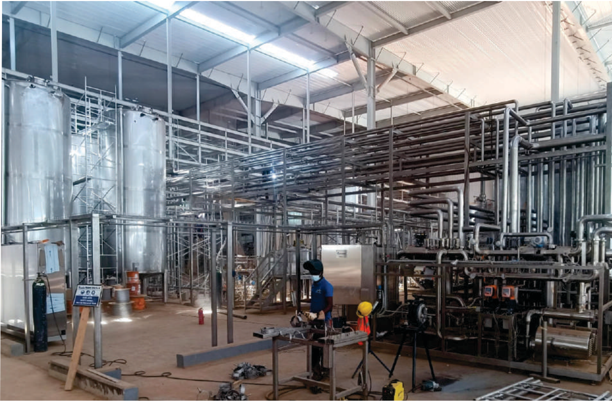
Process Room Installation
