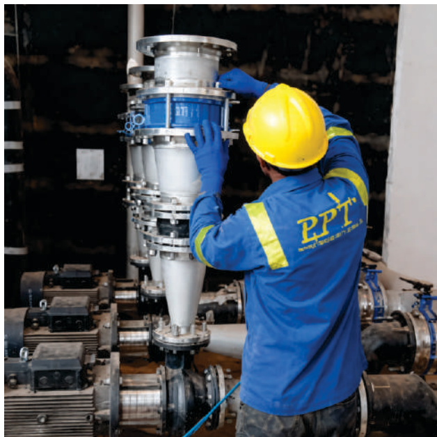
Chilled Water Piping
